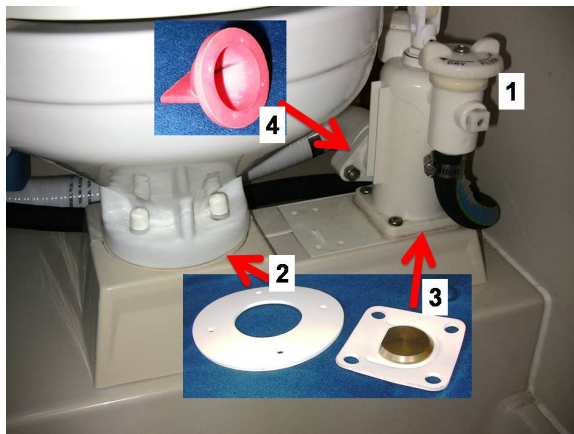
Figure 1: The working parts of a marine sanitation device (Raritan PH-II).
